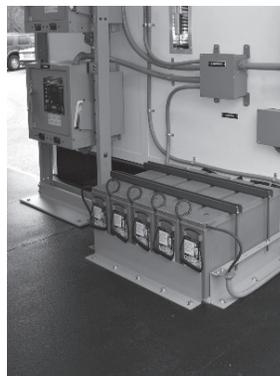
Figure 2b: Five VRLA battery containers on one wall of a trailer. Each has six cells, for a total of 30 cells. The other side of the trailer has 30 more. Combined it is a 60 cell, 120 V string, the most common combination
